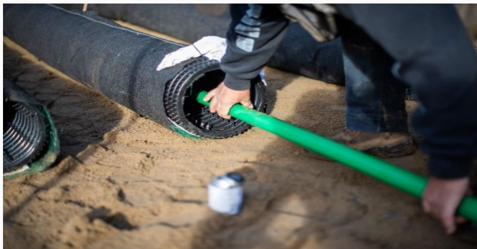
Figure 2: Nested Pipe Configuration, BMEC #23-06-408
