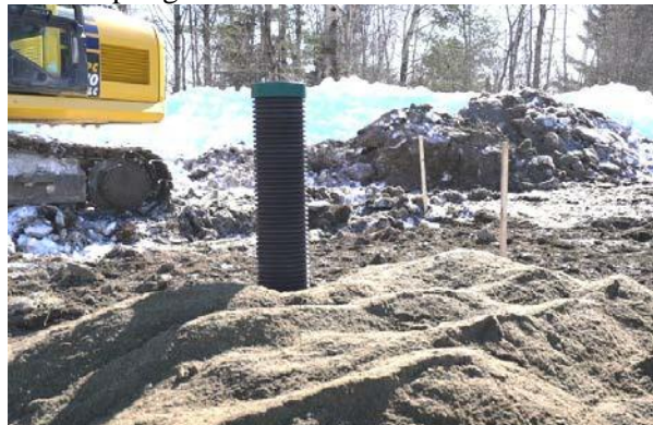
Figure 59. Final installation of the sampling device
