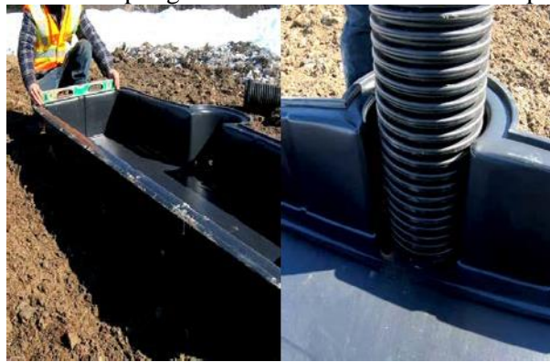
Figure 58. Sampling well installation
