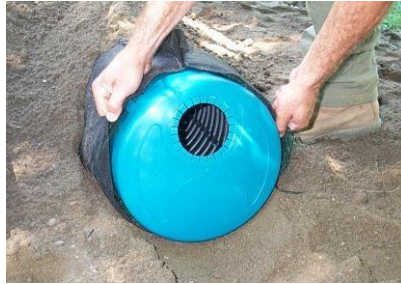
Figure 68. Installation of the Single Offset Adapter
