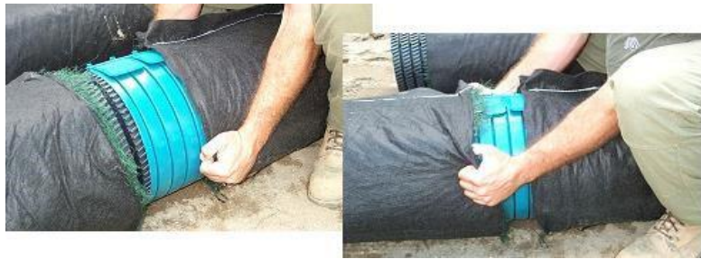
Figure 63. Replacing the geotextile over the couplings
