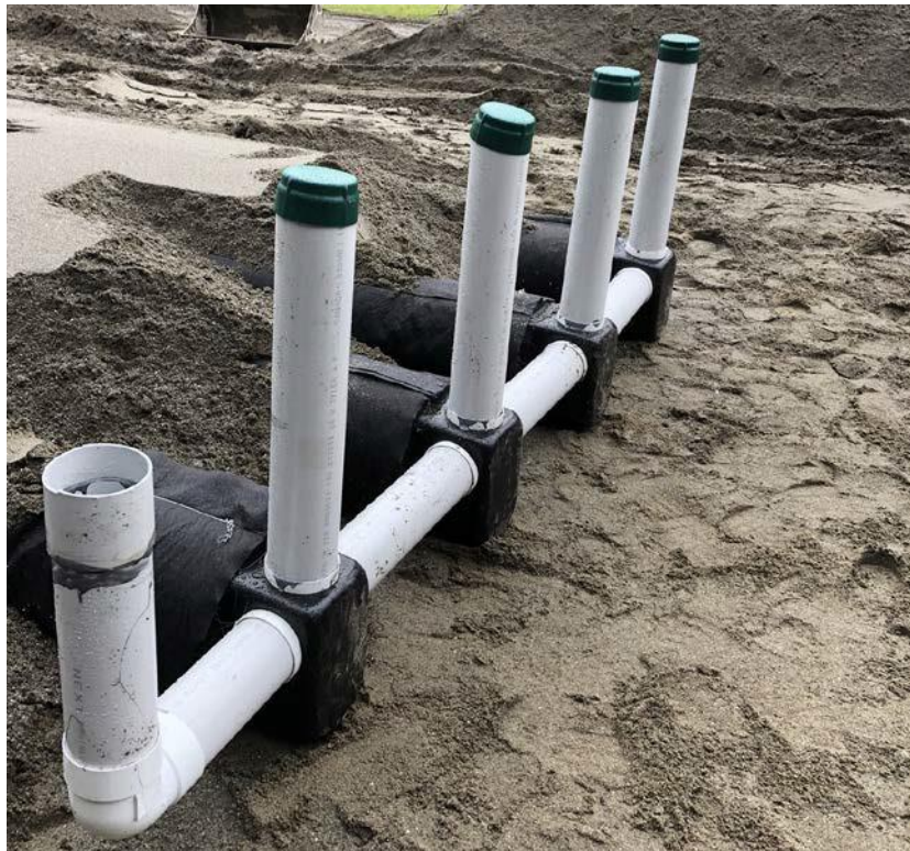
Figure 70. Entry vent on an extremity row
