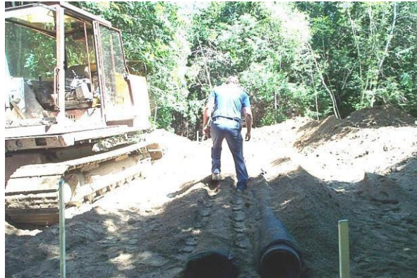
Figure 65. Filling the void around the Advanced Enviro-Septic pipes
