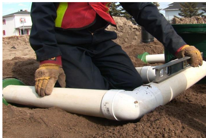
Figure 74. Inlet Pipe sloped toward Advanced Enviro-Septic
