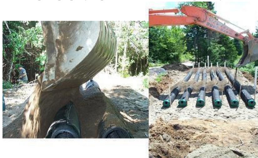
Figure 64. Covering the AES pipes
