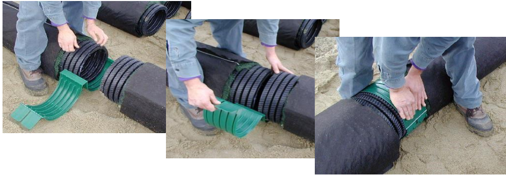
Figure 62. Installation of the couplings
