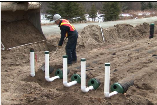
13. Install the piezometers making sure that the horizontal pipe is level.
