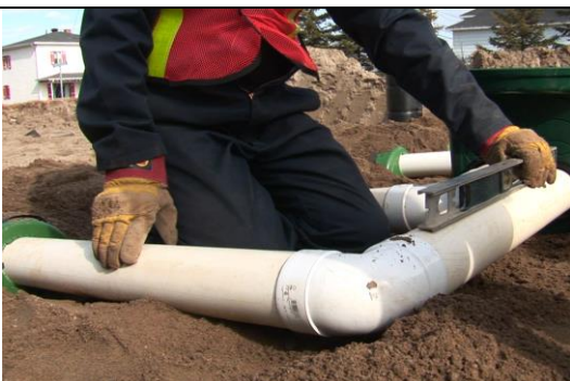
15. Install the distribution box and make sure it is levelled. Install the feeder pipes maintaining a 1% slope toward the Advanced Enviro-Septic® Pipes
