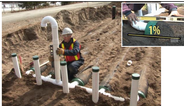
14. Install the ventilation manifold and the entry vent, keeping a 1% slope toward the Advanced Enviro-Septic® Pipes.
