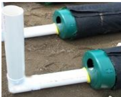
Figure 64 – Piezometer installation
