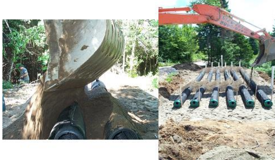
Figure 61 – Covering the Advanced Enviro-Septic® pipes
