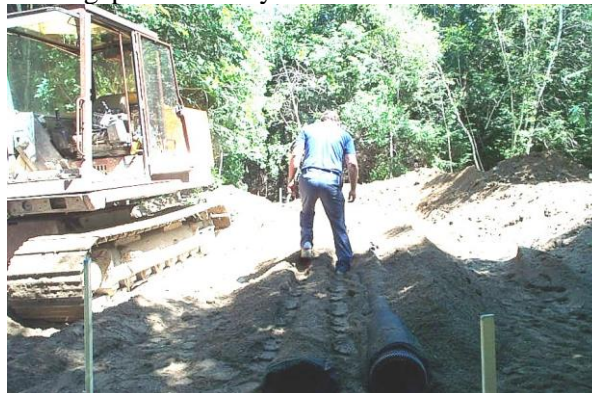
Figure 62 – Filling the void around the Advanced Enviro-Septic® pipes
