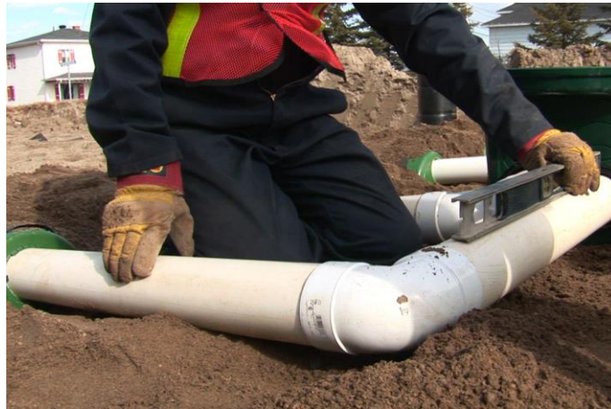
Figure 70 – Inlet Pipe sloped toward Advanced Enviro-Septic®
