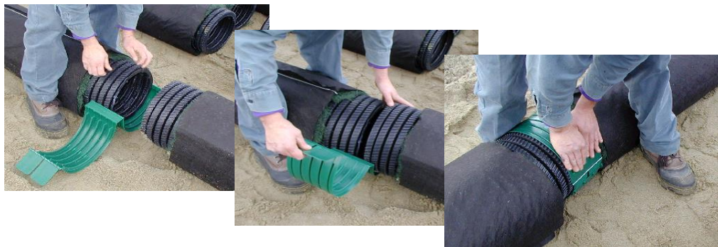
Figure 56 – Coupling Installation
