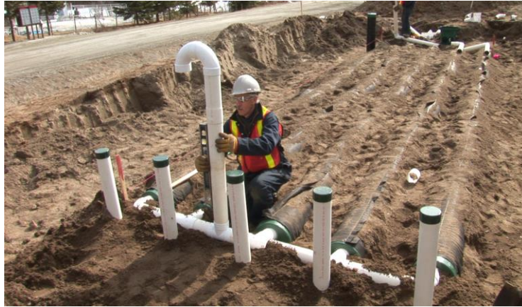
Figure 65 – Aeration pipe and vent installation
