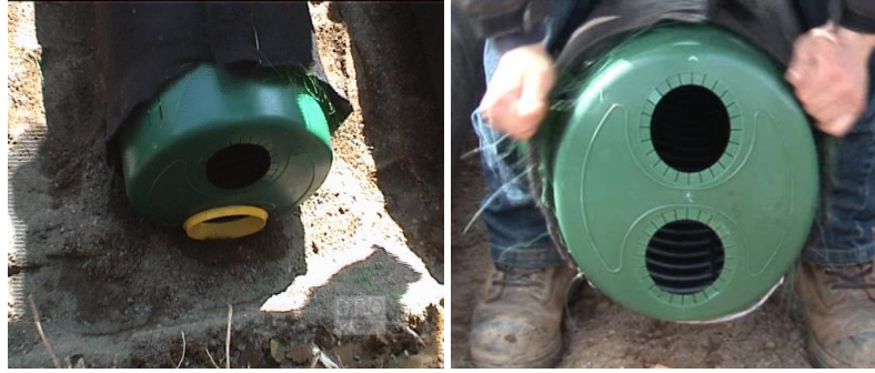
Figure 59 - Installation of the double offset adapter (old and new style)
