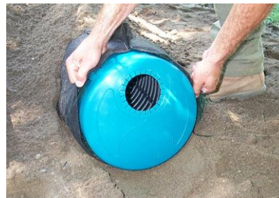
Figure 58 – Installation of the Single Offset Adapter
