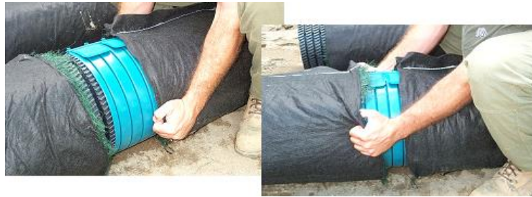
Figure 57 – Replacing the membranes over the coupling
